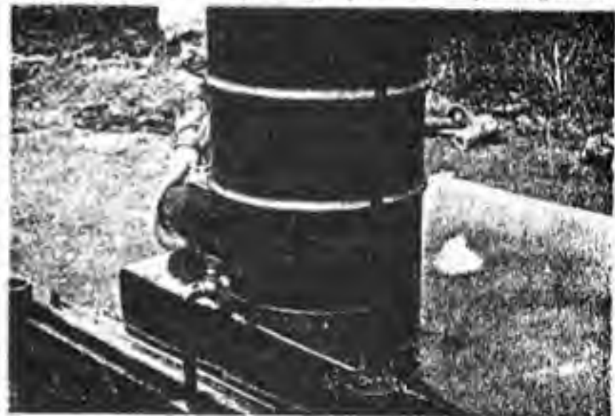
ILLUSTRATION 11. The metal barrel feeding-unit of the "Apolo Spessard-Hydroponicum" at Rio de Janeiro, Brazil, in the course of construction, as modified and constructed by Mr. A. S. Jacobsen, the ingenious gentleman shown in the photograph. Special precautions were taken in this construction to avoid growing difficulties due
